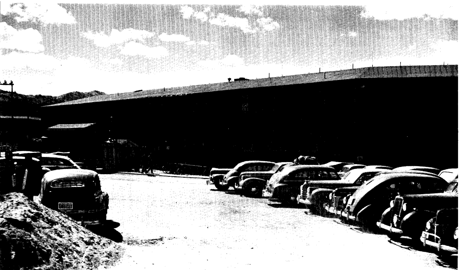
technical area. Gamma building, below and at right above, wrapped around and obscured red Ashley Pond.
